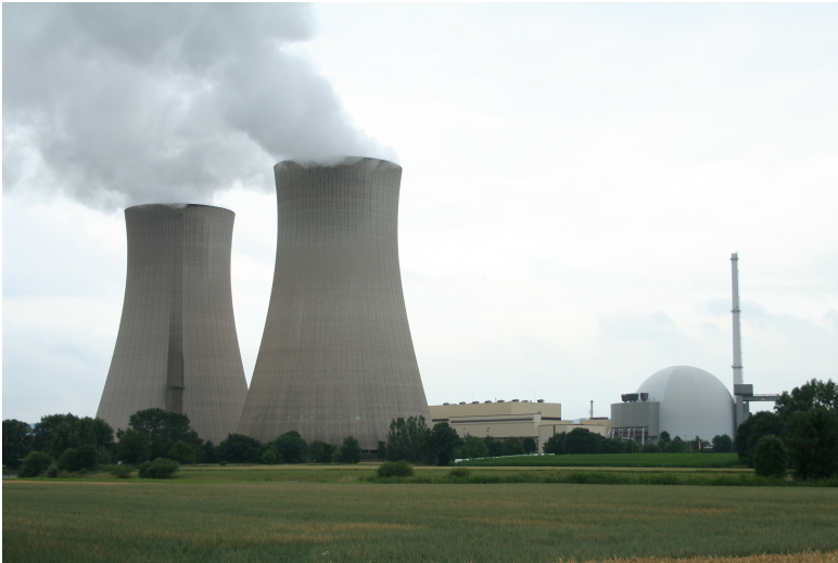
Here is a nuclear power plant in Germany. The white dome is where the uranium atoms are split inside the nuclear reactor. The large towers release steam created when the heat of the reactor boils water.
